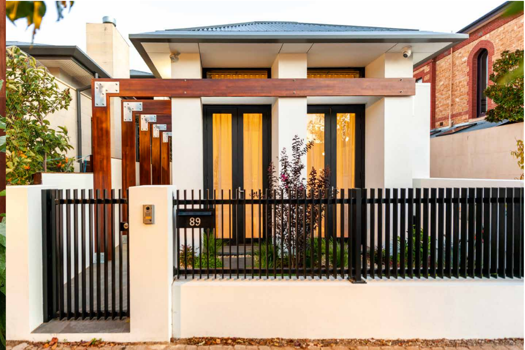
Above and opposite page: Merbau beams have been used to create an architectural canopy, defining the pathway from the gate to the front door.
